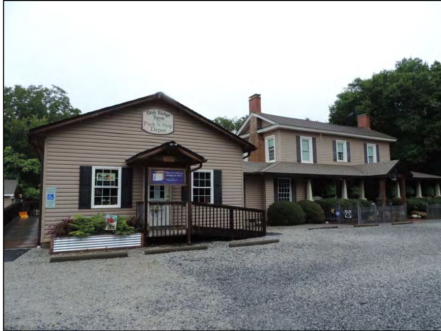
Figure 6: Facing northeast along Seigler House's south façade
