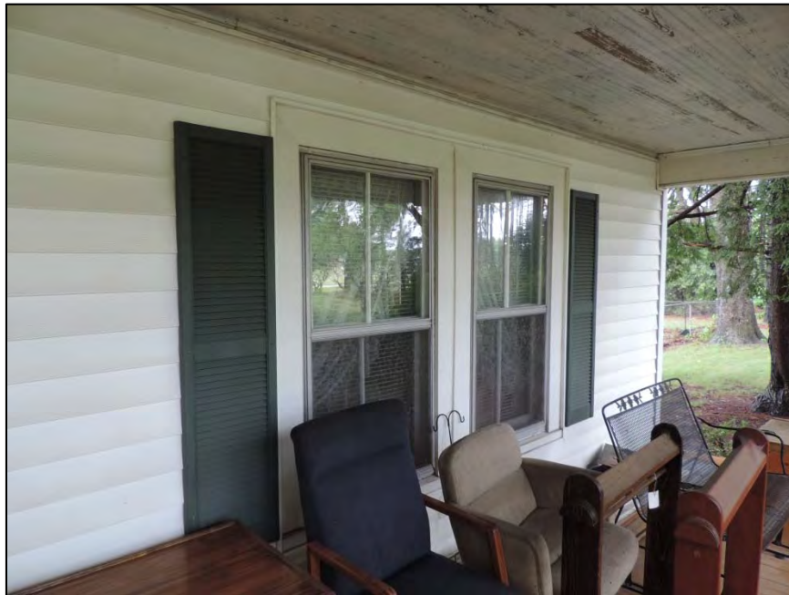
Figure 33: Brumley House, window detail
