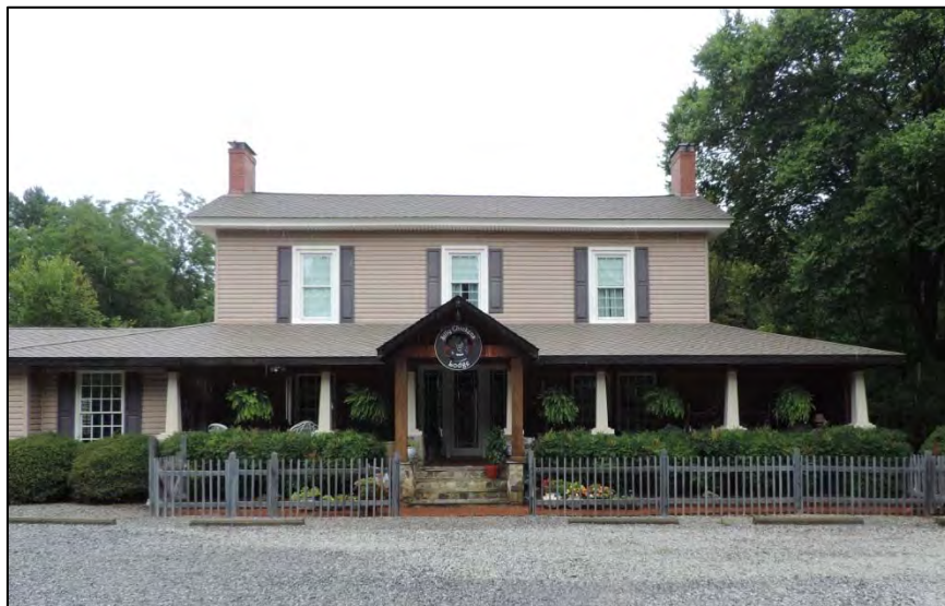
Figure 7: Facing north to Seigler House's original mass
