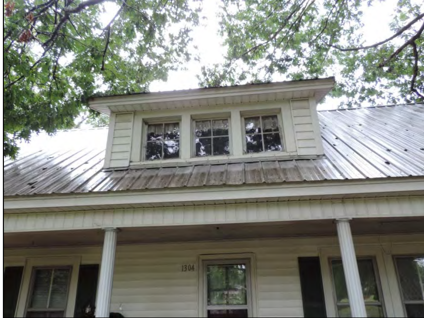
Figure 34: Brumley House, dormer detail
