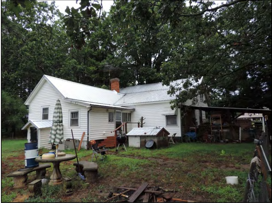
Figure 38: Brumley House, facing northwest to rear, south elevation
