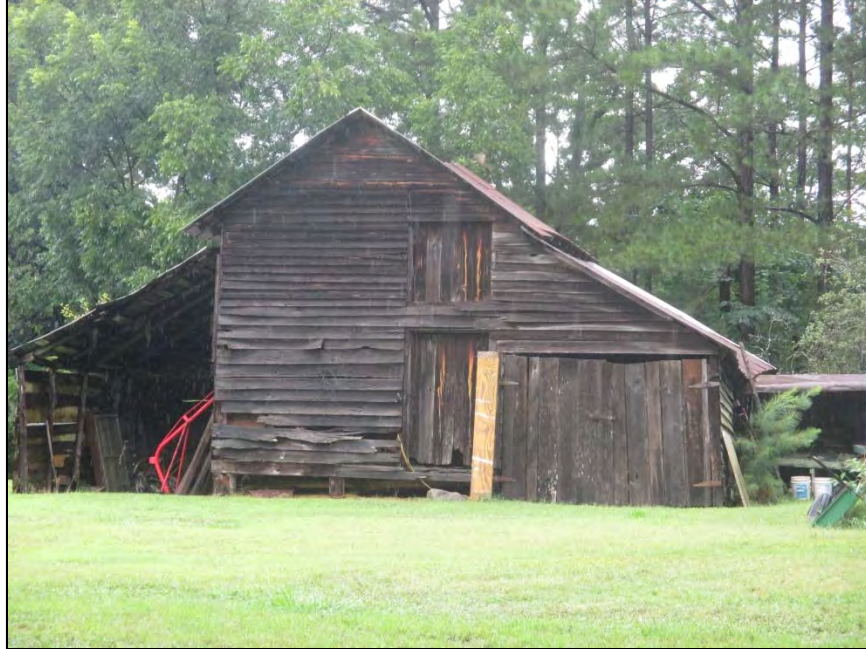
Figure 41: Brumley House, facing northwest to large barn
