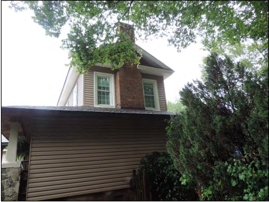
Figure 12: Seigler House, east side elevation (see also Fig. 6)
