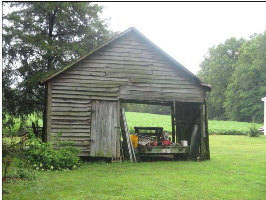
Figure 42: Brumley House, facing southwest to small barn
