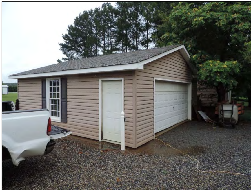
Figure 18: Seigler House, facing northwest to southern detached storage building
