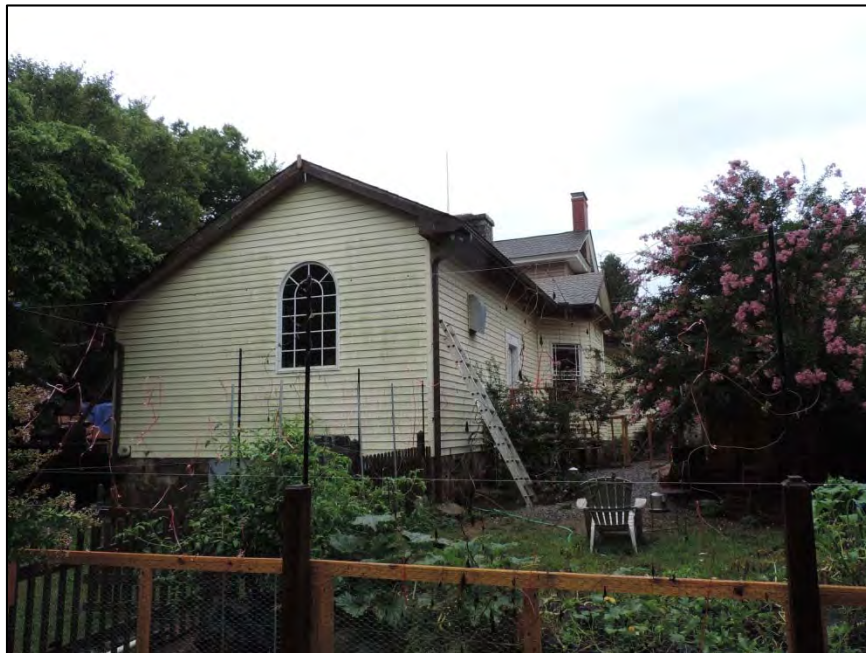
Figure 16: Facing south to Seigler House's rear north elevation and along rear addition's west side elevation
