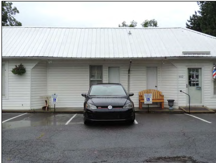
Figure 66: Staton Store, detail of central storefront
