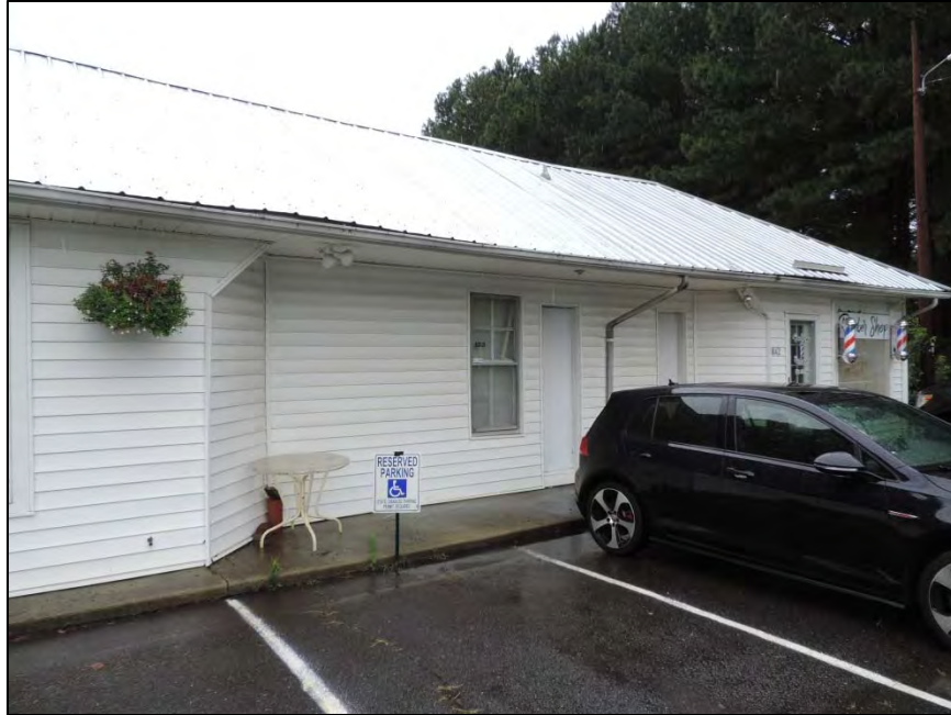
Figure 67: Staton Store, detail of central storefront
