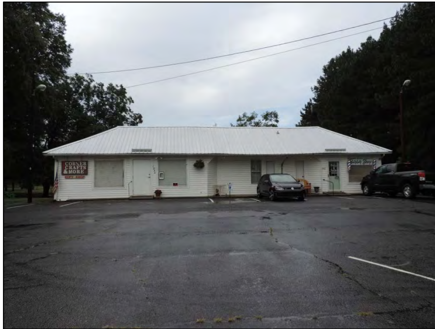
Figure 64: Facing south to Staton Store from Landis Highway
