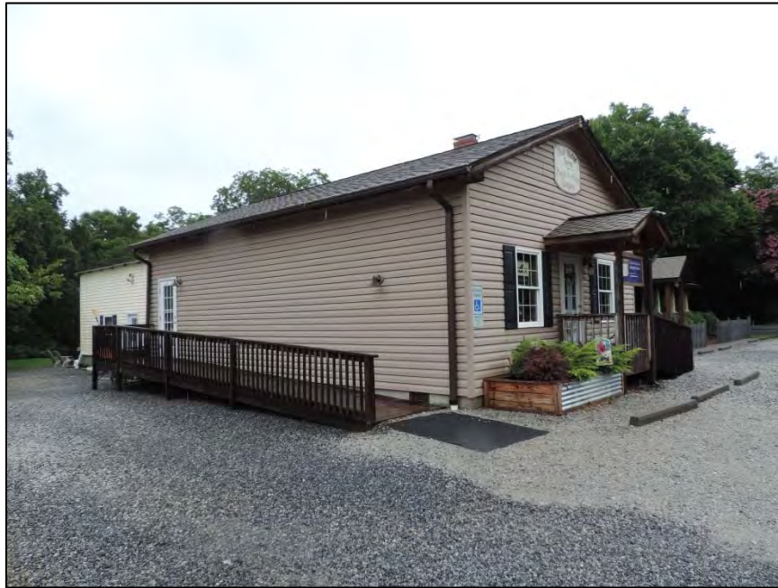
Figure 14: Seigler House, west side elevation of additions
