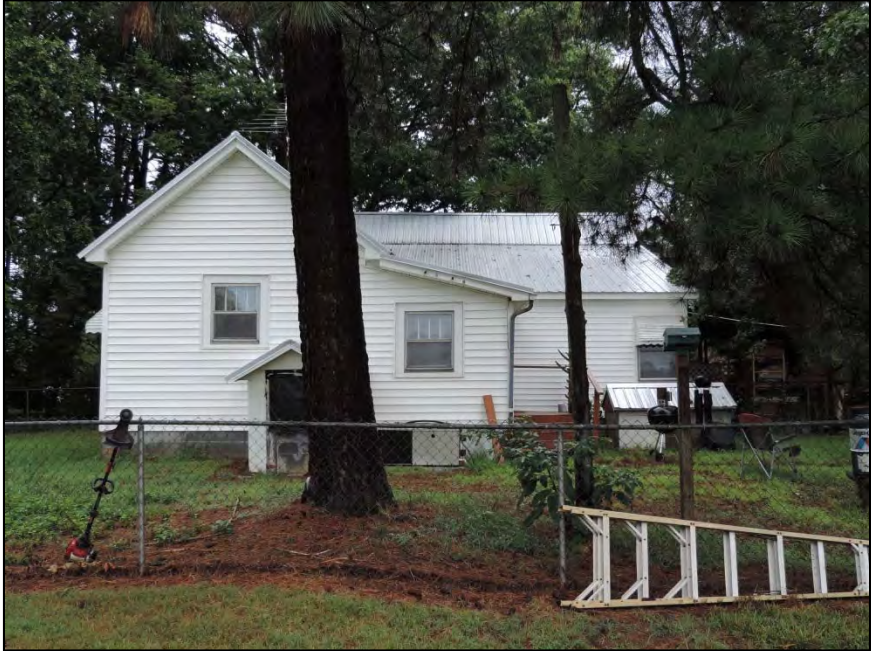
Figure 39: Brumley House, rear south elevation
