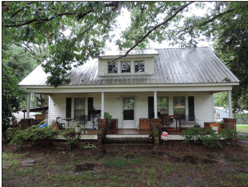
Figure 31: Facing south to Brumley House
