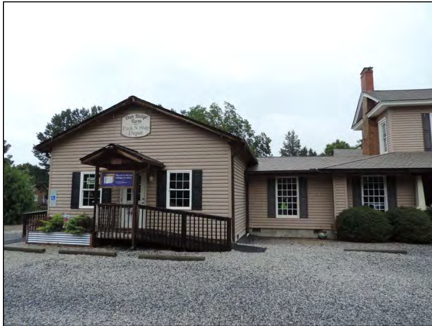
Figure 10: Facing northwest to Seigler House's non-historic shop addition and hyphen
