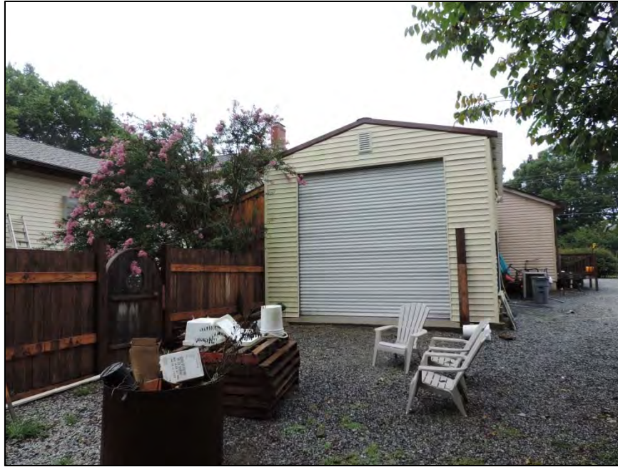
Figure 17: Seigler House, facing south to rear elevation of metal-clad addition
