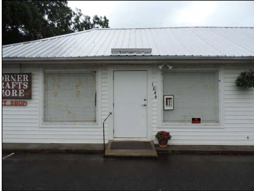
Figure 65: Staton Store, detail of east storefront
