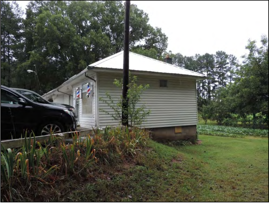
Figure 70: Staton Store, west side elevation
