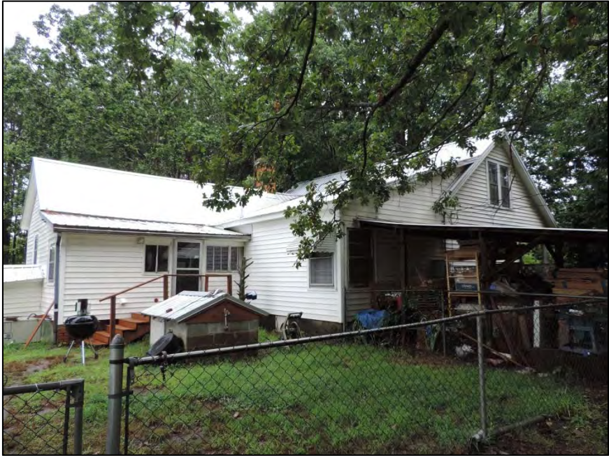
Figure 37: Brumley House, facing northwest to east side elevation and rear, south elevation
